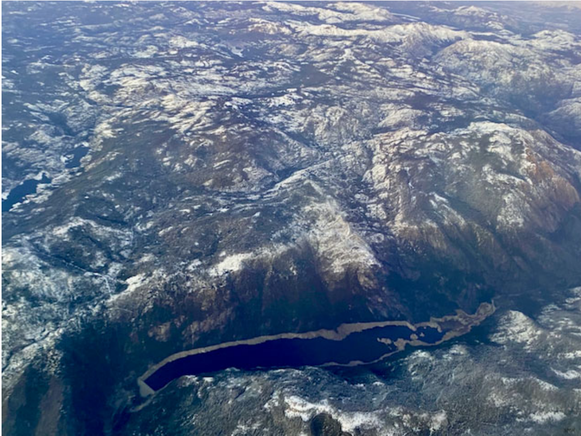
The site of the proposed battery project - Salt Springs Reservoir (center) and the Bear River Reservoirs (upper left) December 2021
